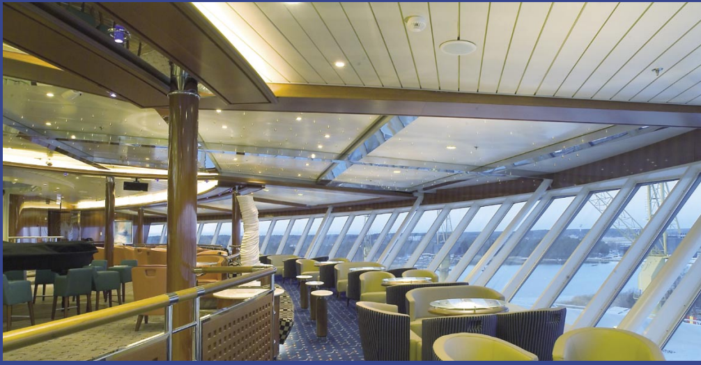
Observation lounge KS-200 panels and metal beams
